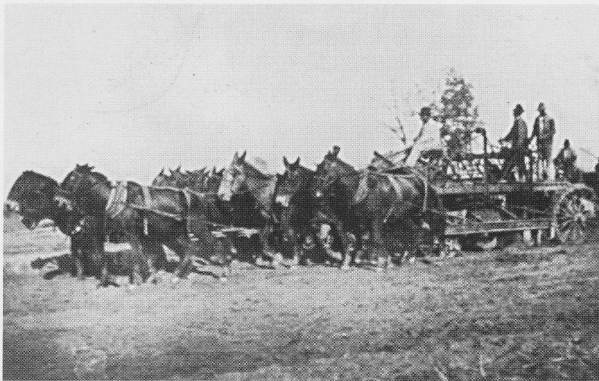
Earth moving machinery, mules and men work on the levee in 1906. Courtesy of the Walters-Boyd Family Papers at the Delta State University Archives.
